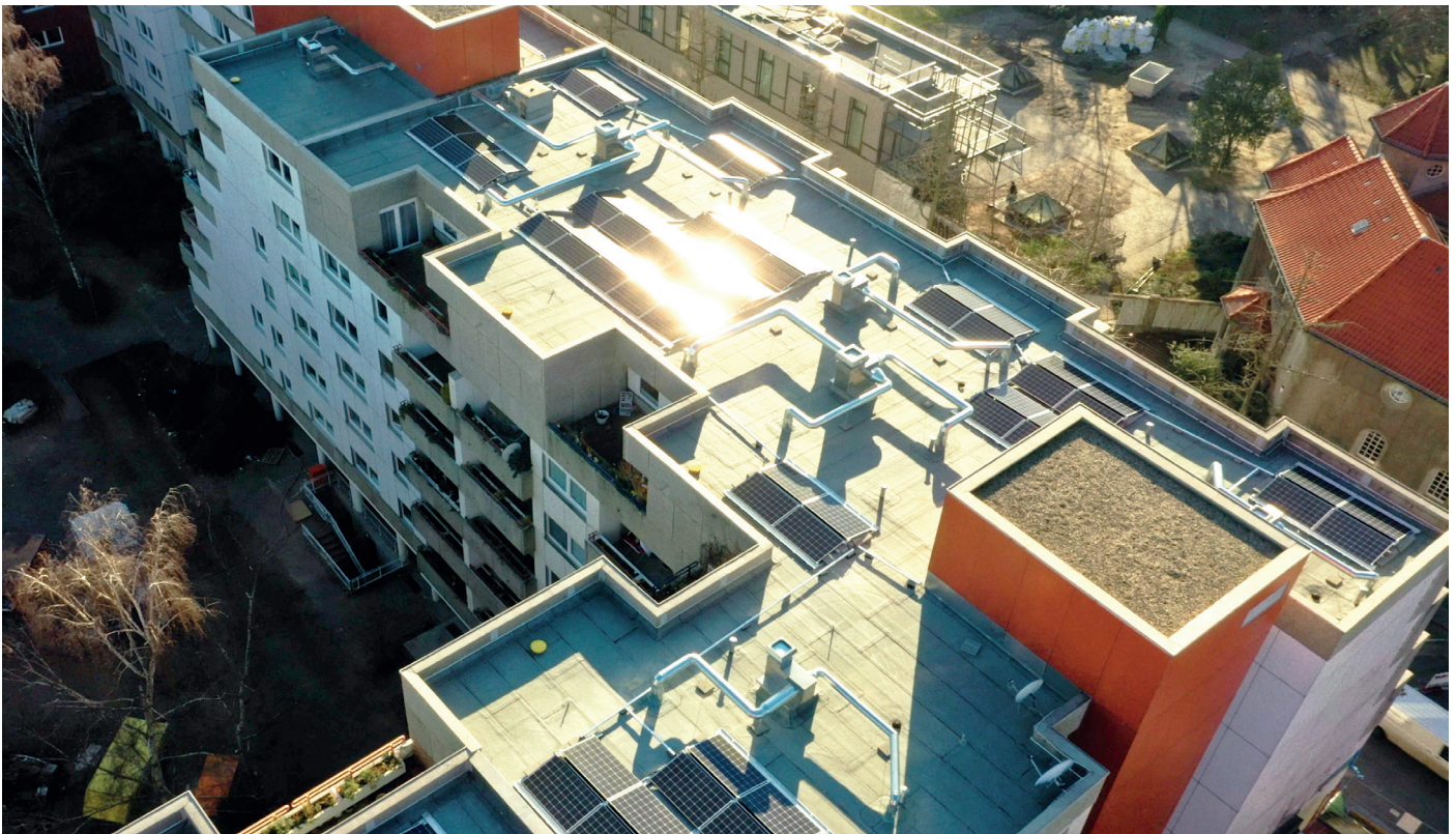
Despite comprehensive ventilation technology on the roof, the system on Adolfstraße 3 generates over 50 kWp. (photo)
